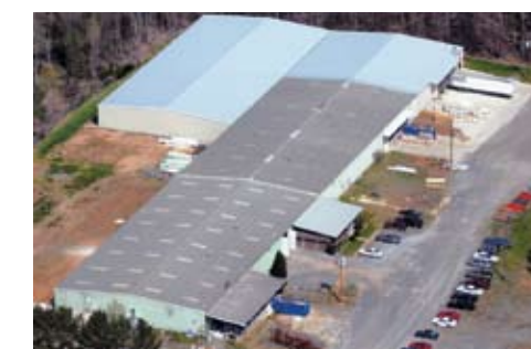
AFCO Architectural Products Pell City, AL
