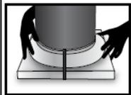
8. Use a high quality caulk to fill gaps where the capital and the base meet the column.
