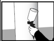
*Finishing instructions: Prepare the column, capital and base for painting by sanding with 100 grit sandpaper or a sanding sponge. Follow the paint manufacturer's instructions for proper surface preparation. Paint with high quality latex or oil based paint.*
