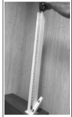
2. When the final position is determined for the post, mark the hole locations of the four 3/8" diameter mounting holes provided on the base and remove the post assembly. Drill the marked locations into the decking and reinforcement using the proper size drill required for the fasteners being used.
