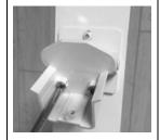
7. Align the Bottom Rail Hinge Assemblies (D) so they are facing parallel to each other, and measure the distance between upper and lower Bottom Rail Hinge Assemblies (D) previously mounted on the posts in step 5.
