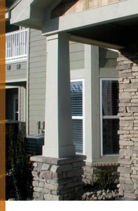
Components designed to center wrap around a nominal 4″ X 4″ wood post.
