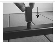
4. Confirm the length of the glass infill being installed and subtract that dimension from the length of the bottom rail cut in step 1, divide that difference by 2. This will be the length of the required insert. Locate the painted Glass Rail Insert (K) and cut /if required/ 4 pc provided to the calculated dimension, these will be used for the bottom rail, and top rail.
