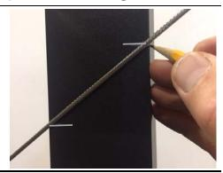
13. Transfer marks from step 12 to both the upper and lower side of the intermediate post. Drill a pilot hole using a (5/32) drill bit in the center of the post at those marks. Using the Installation Tool, align the hole drilled with the top "cable hole" on the tool, locate the lower "cable hole" on the tool and drill holes down the post on opposite sides for the required amount of cables being installed. Once pilot holes are drilled, or marked, drill out each hole to a 1/4" diameter.
