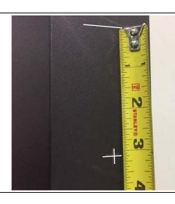
10. Using the Installation Tool, align the holes drilled in step 9 with the top "cable hole" on the tool, locate the lower "cable hole" on the tool and drill holes down the post on opposite sides, repeating for the required amount of cables being installed using the Installation Tool for correct spacing.
