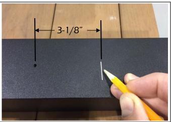
2. From that reference mark in step 1 measure down towards the base of the post 31" for 36" height rail, and measure down 37" for 42" height rail.
