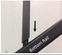
19. At the point where you installed the support block connectors (step 16), carefully measure the distance from the underside of the bottom rail (B) to the stair tread. Cut support block material (K) to fit. Slip support block over support block connectors (L). Slide the rail back into place and make certain the rail is plumb.
