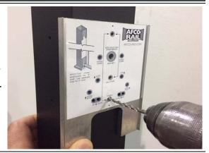
11. If installing an intermediate post on stair treads, locate post in desired position and ensure the minimum clearance to the top of the post is achieved from the top side of the Bottom Rail (B) to the top of the post the same as in step 4.
