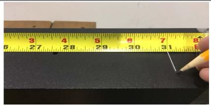
3. Place upper post in the desired position with reference marks facing towards the stairs. Lay the Bottom Rail (B) on the stair-nosing from top to bottom, and adjacent to the post. Align the lower reference mark from step 2 with the top edge of the bottom rail. (Post can be mounted with reference line higher than the top of the bottom rail if desired) Post should not be mounted with reference mark below the top side of the bottom rail.
