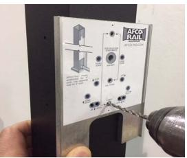
14. From the center of the top hole drilled, on both sides of the post, measure up 3-1/8" and place a mark across the post. Align Screw holes in the Upper and Lower Saddle Brackets (C&D) on the marked lines on the posts. Make sure the brackets are centered on the posts. Mark the screw hole locations with a pencil.
